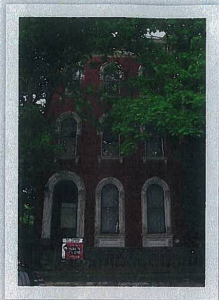
ABOVE & BELOW: Contractor Todd McFarland spent three years restoring this Italianate town house in Cincinnati's resurgent Over-the-Rhine Historic District (believed to be the largest urban historic district in the country), netting him a local preservation award. RIGHT: Boston's Beacon Hill is Massachusetts' oldest historic district, and homeowners there are held to a strict set of guidelines—those wanting to replace missing architectural features, for instance, must provide evidence of the originals.
